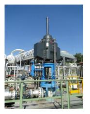
Line Shaft Pump (LSP) Setting depth: 350 m Power consumption: 160 kW Oil lubricated LSP Wellhead pressure: 22.5 bar
