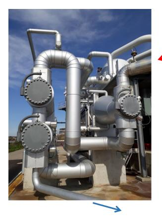
Na-Ca-Cl fluid with a TDS of about 100 g/L and a Gas Liquid Ratio of 1 (86% CO<sub>2</sub>) The plant has an installed gross capacity of 1.7 MWe, and a annual baseload factor > 90%
