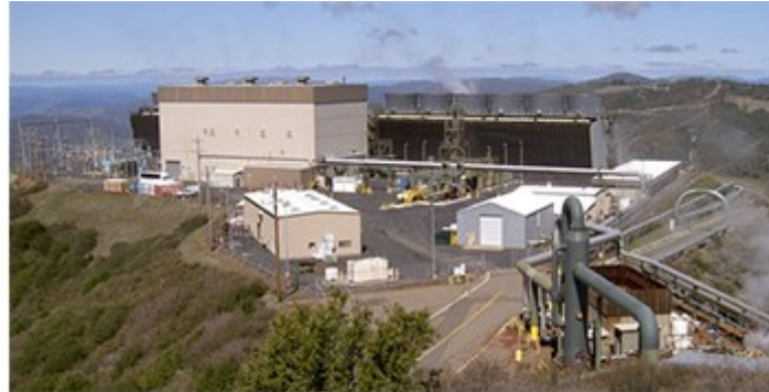
The Sonoma Calpine 3 geothermal power plant at The Geysers field in the Mayacamas Mountains of Sonoma County, Northern California. (Licence: CC0 1.0)
