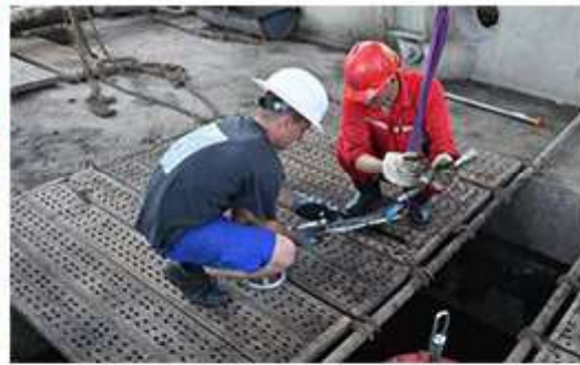
Installation of the geophone chain (view from the well head).
