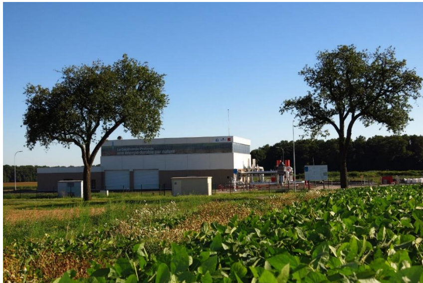
Figure 4 The recent geothermal plant of Rittershoffen producing heat at high temperature ( >160^{\circ}\text{C} on surface) in the Upper Rhine Graben, source ES
