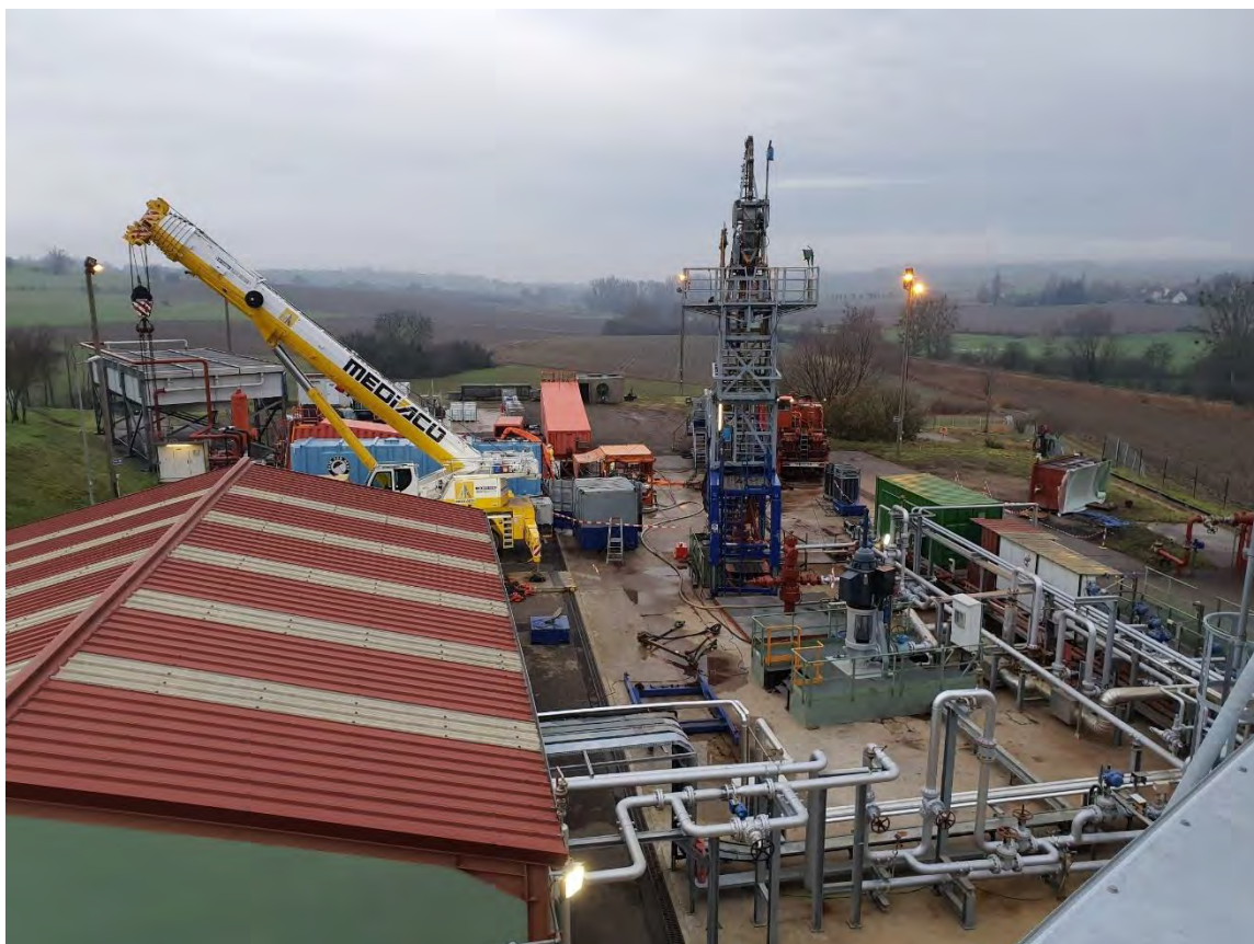
Figure 33: Picture of Soultz site after rig up of the stimulation equipment.
