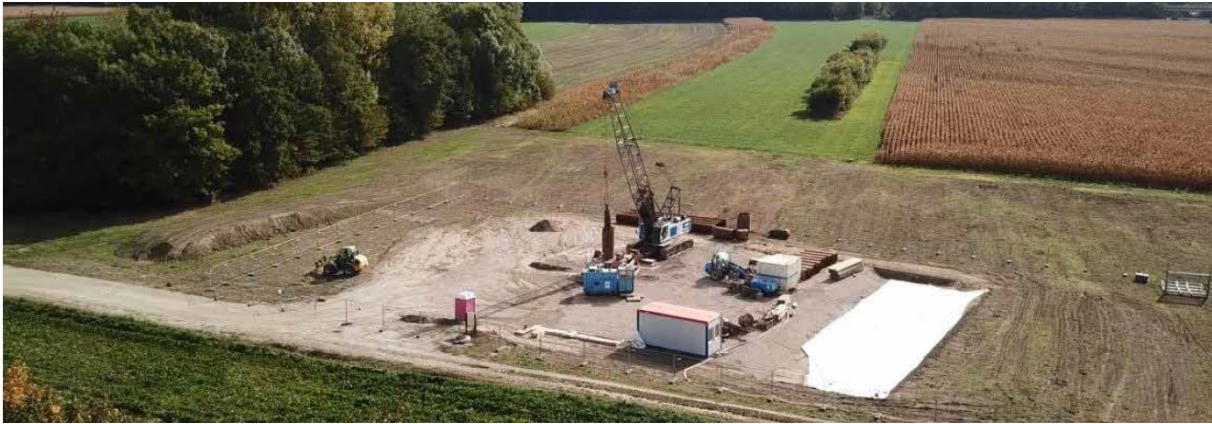
Fig. 39 Study site drilling platform ©és
