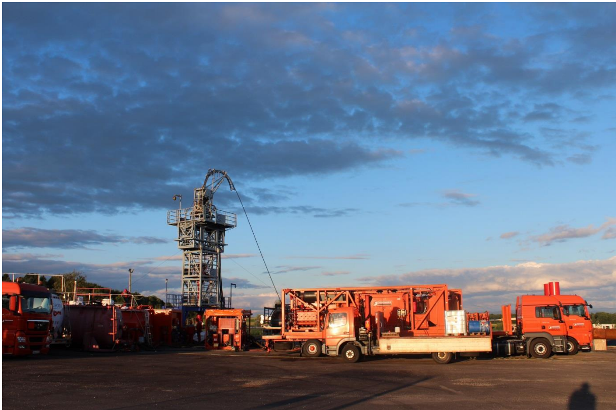
Fig. 1 Chemical stimulation operation at Rittershoffen geothermal site (France). ©és
